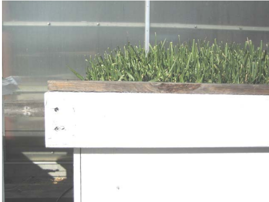
Fig. 6: The green roof.
