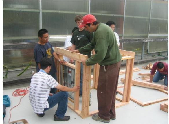
Figure 4: Construction of the Test Cells at the Lyle Center
